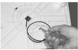
2. Remove necessary knockouts and fasten back plate to j-box.
