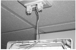
3. Remove hole plug and dress leads through housing wire channel. Snap exit housing onto canopy.
