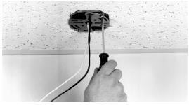
Remove face place. Connect jumper leads (provided) to AC input leads in j-box. Fasten j-box bracket to j-box.
