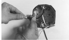
Remove faceplate. Connect installation supply leads (provided) to AC input leads in j-box. Remove face plate and back plate from housing.
